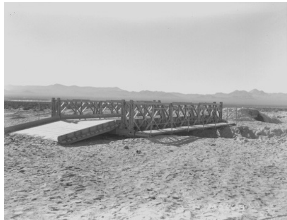
Bailey Bridge, Position #1
